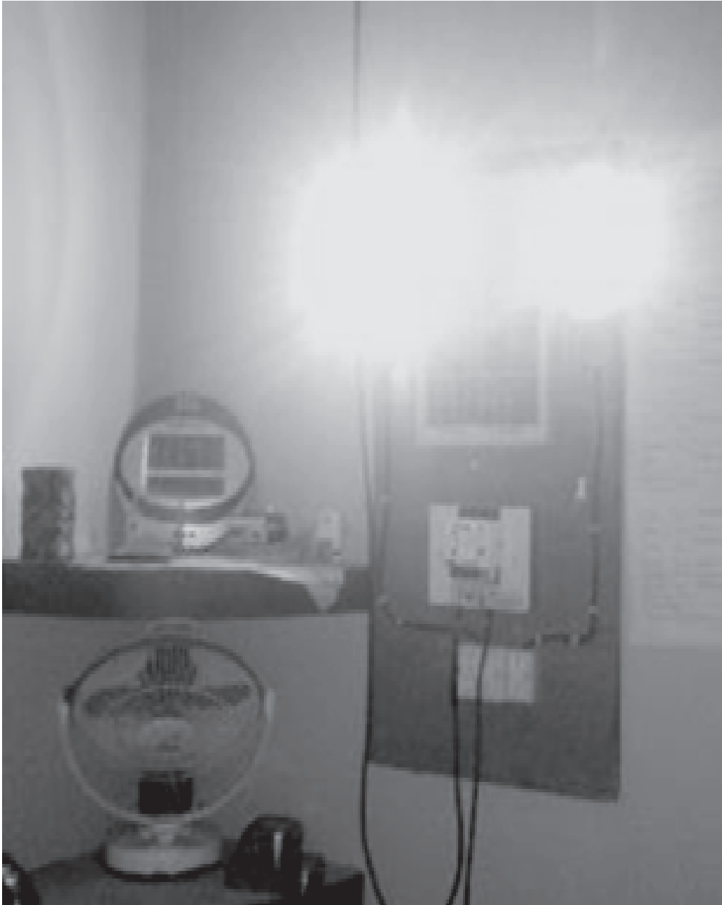
Figure A1. Normal Solar Home System and its Various Components (SEWA Bharat Office at Munger in Bihar)
